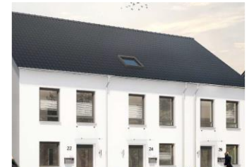
Construction apartments, Berlin/Brandenburg (Germany)
