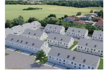
Construction terraced houses, Britz (Germany)
